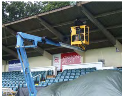
Installing the new sound system
