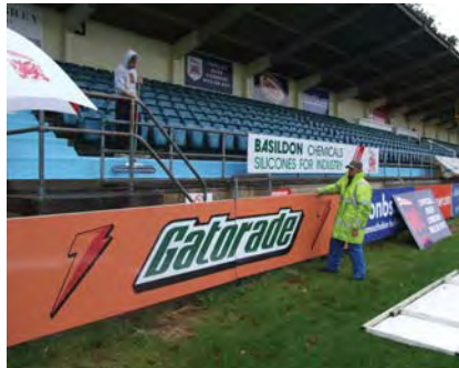
New and updated touchline hoardings are installed
